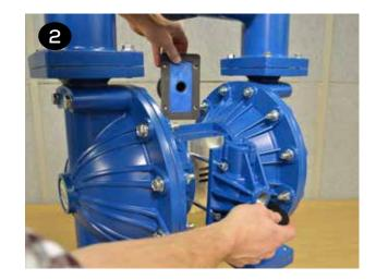
• Place the new gasket (item 38) on the air valve (item 3) and ensure the slots in the gasket align with the slots in the air valve and valve plate (item 10).
